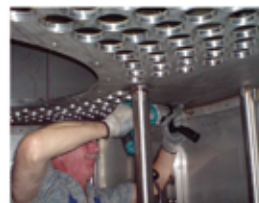
Heat exchanger being built
